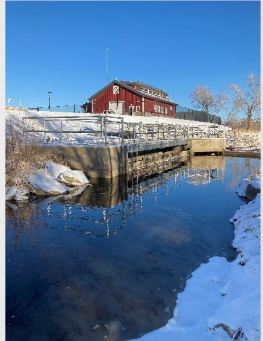
Plum Creek Diversion and Pump Station
