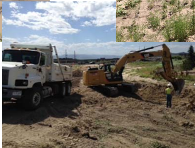
Stormwater crew removing excess sediment
