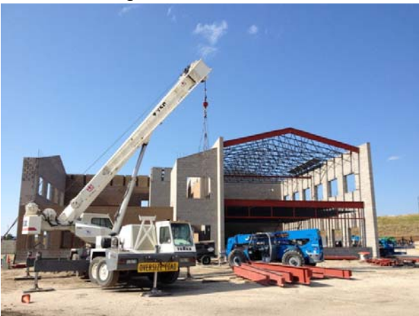
Steel installation in progress
