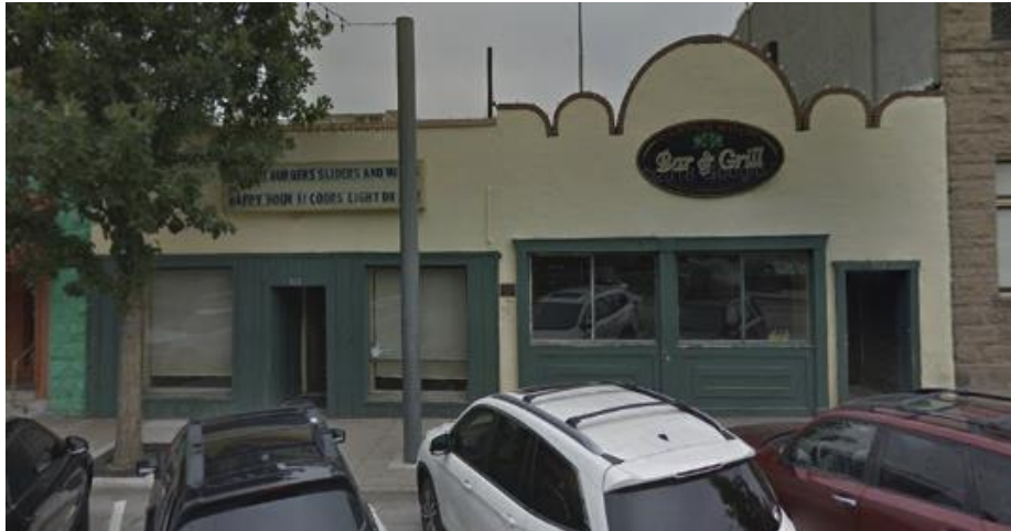
Street View of Existing Wilcox Street Façade
