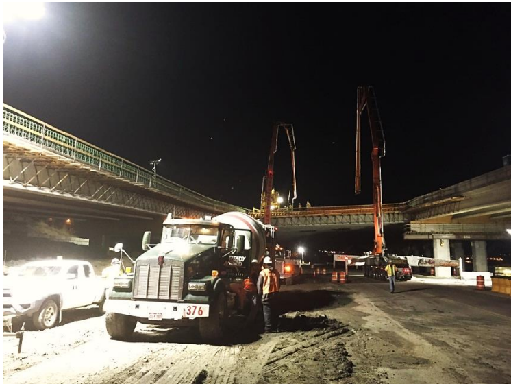
Concrete Placement of the Bridge Deck US 85 (night work)
