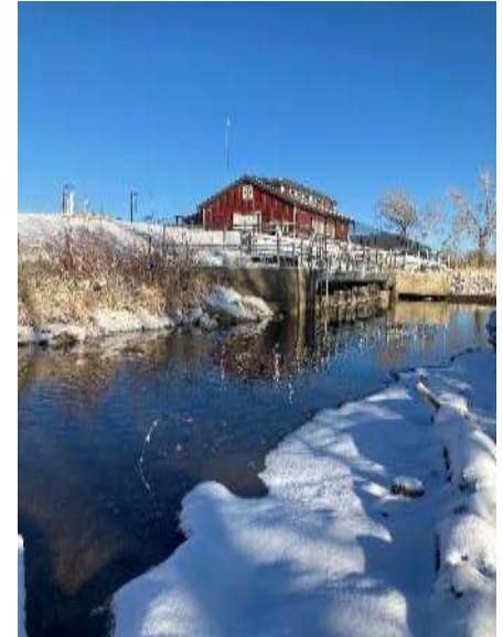
Plum Creek Diversion and Pump Station
