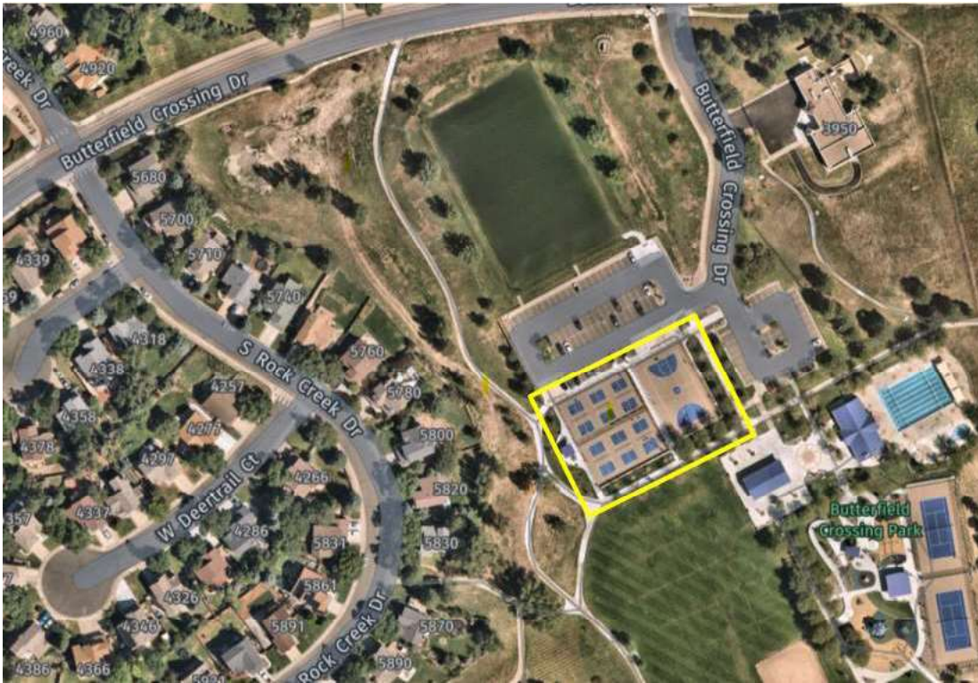
Sport Court Location at Butterfield Crossing Park | Post-renovation, August 2023
