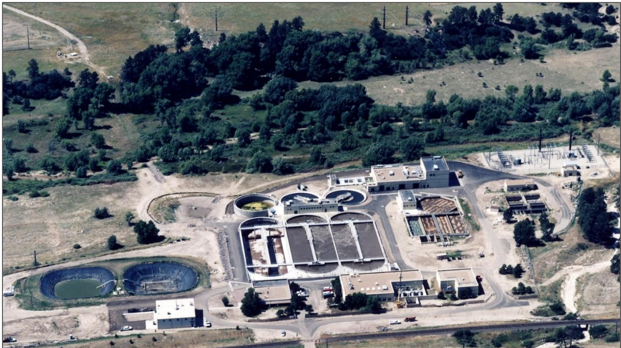
Figure 13: Aerial View of the Plum Creek Water Reclamation Authority Facility (Plum Creek Water Reclamation Authority, 2017)
