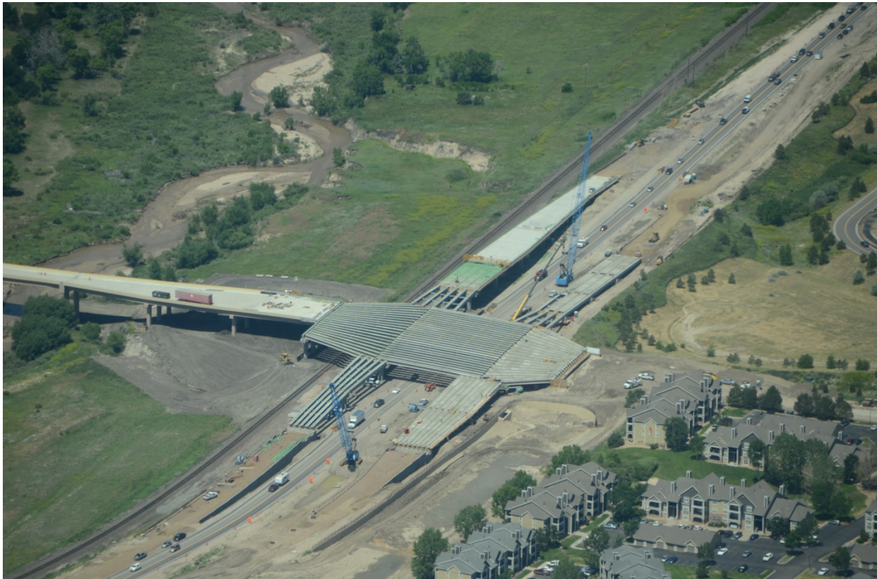
FINAL GIRDER PLACEMENT FOR THE NORTH MEADOWS EXTENSION
