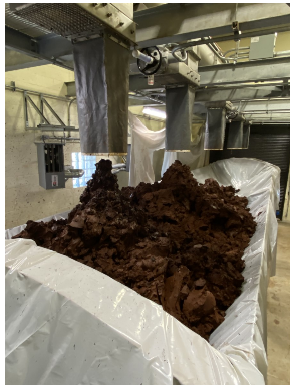
Treatment residuals loadout at PCWPF.
