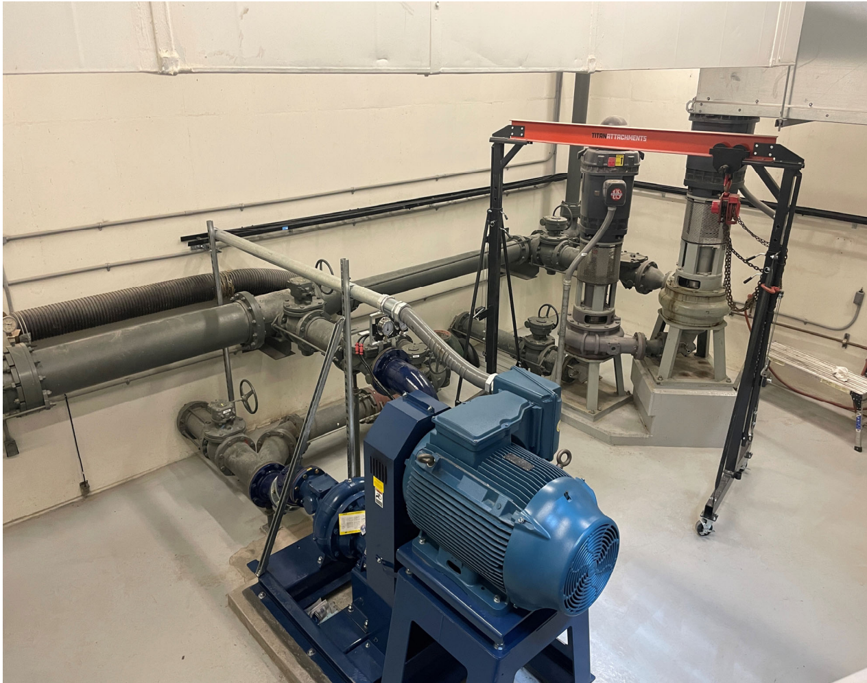
Castle Oaks Lift Station - New pump installer
