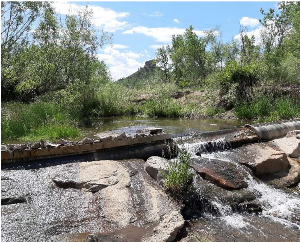
CR-1 Diversion structure along East Plum Creek
