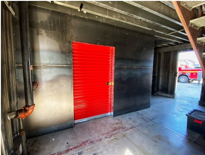
New door at FTC
