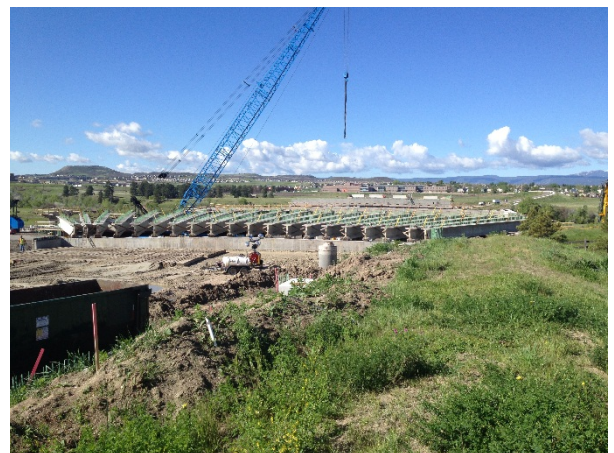
North Meadows Extension in progress
