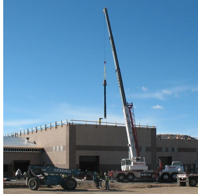
VT Pump install, 2012
