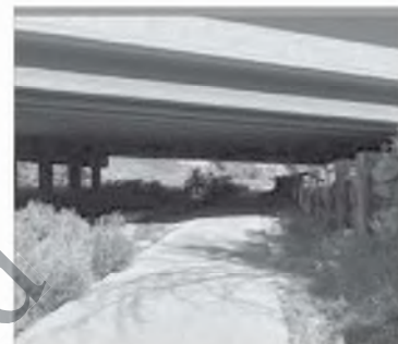
Existing retaining wall upstream of I-25 Bridge over East Plum Creek.
