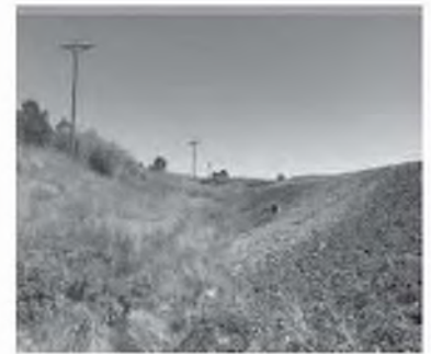
Ditch between BNSF and Prairie Hawk Drive.
