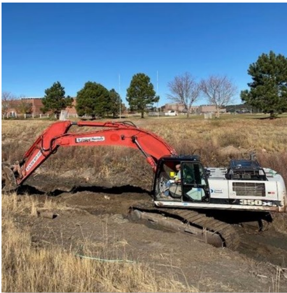
Linkbelt Excavator Conducting Storm Pond Remediation Operations
