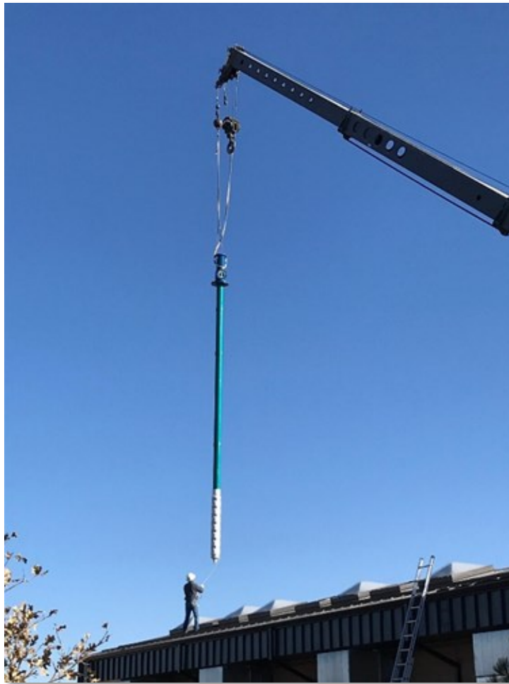
Green Zone Pump Installation
