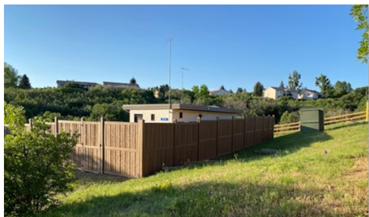
Newly Constructed Fencing at Enderud Well House
