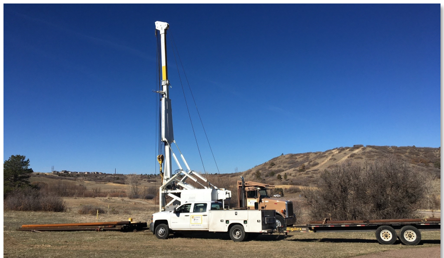
Colorado Pump pulling equipment at CR-72R
