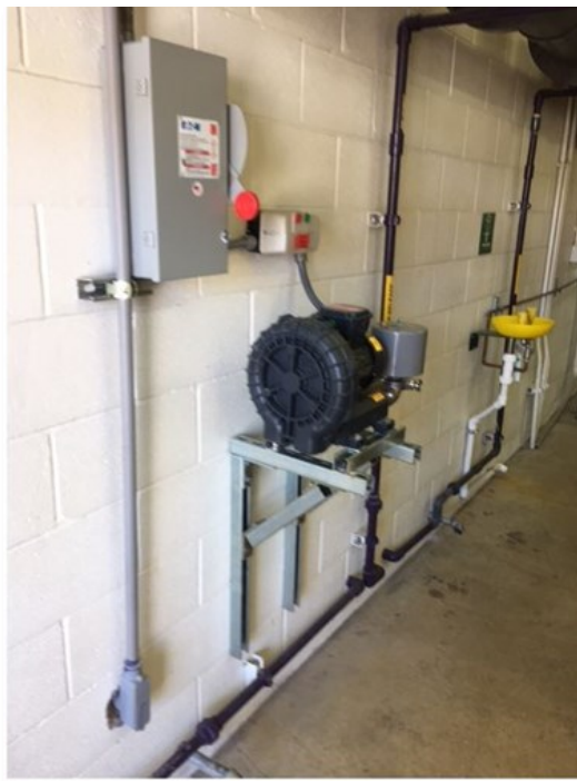
Wet Well Wizard Blower and Ejector System
