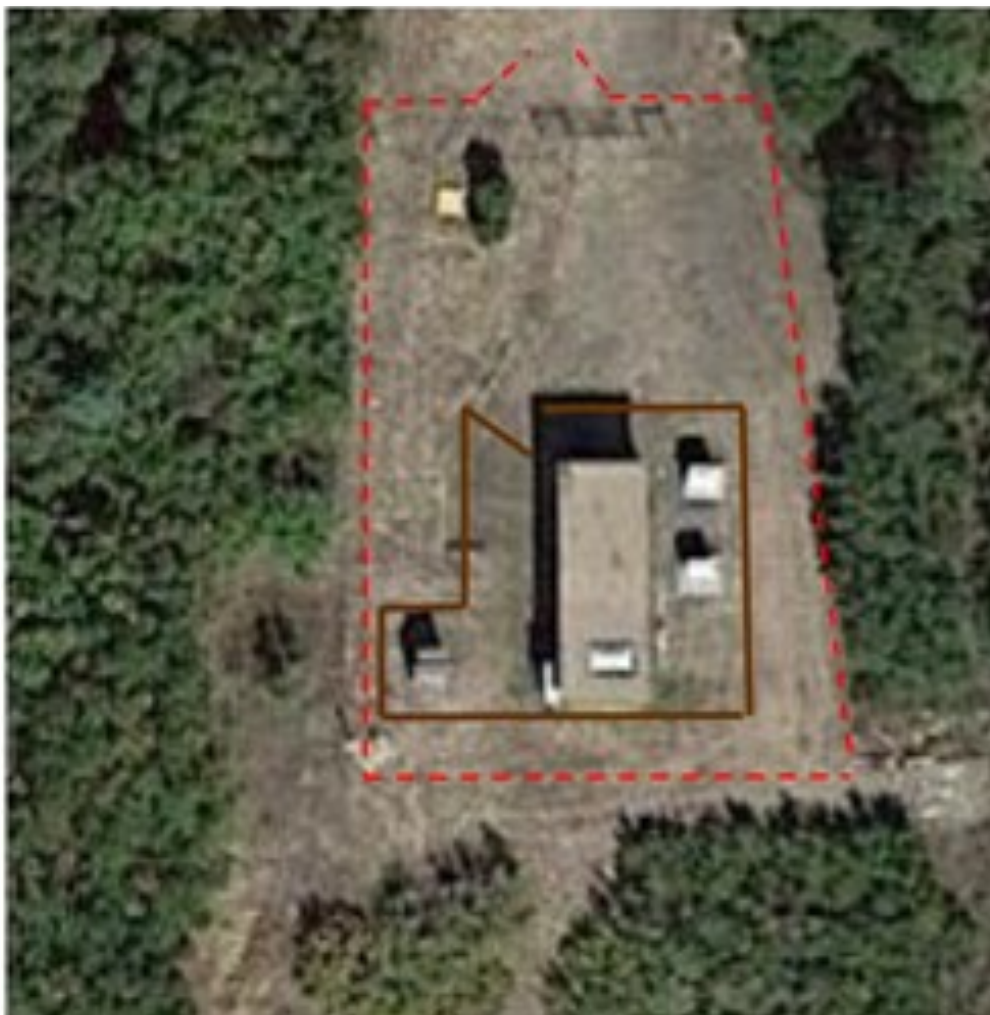
Fencing at 4286 Hidden Gulch Rd., Castle Rock
