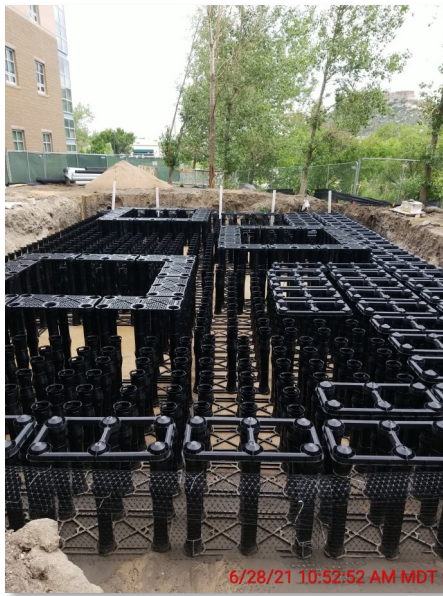
Silva Cells Under Construction
