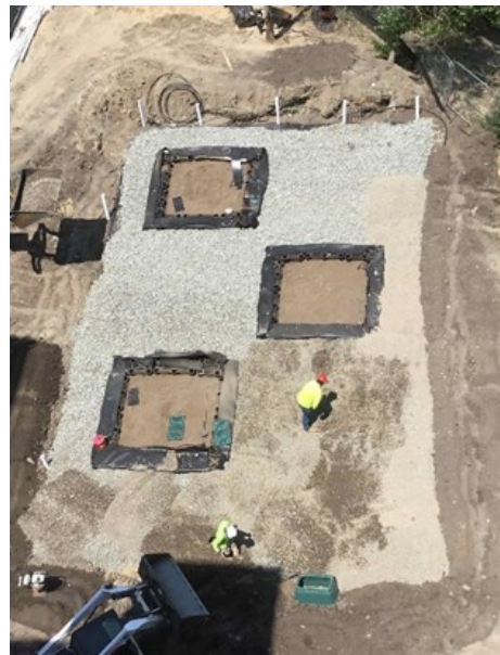
Porous Paver Subgrade Over Silva Cells
