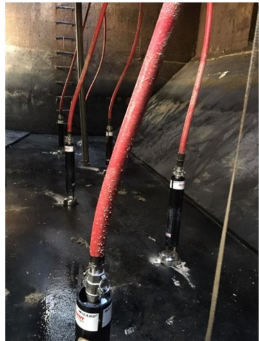
Wet Well Wizard Blower and Ejector System
