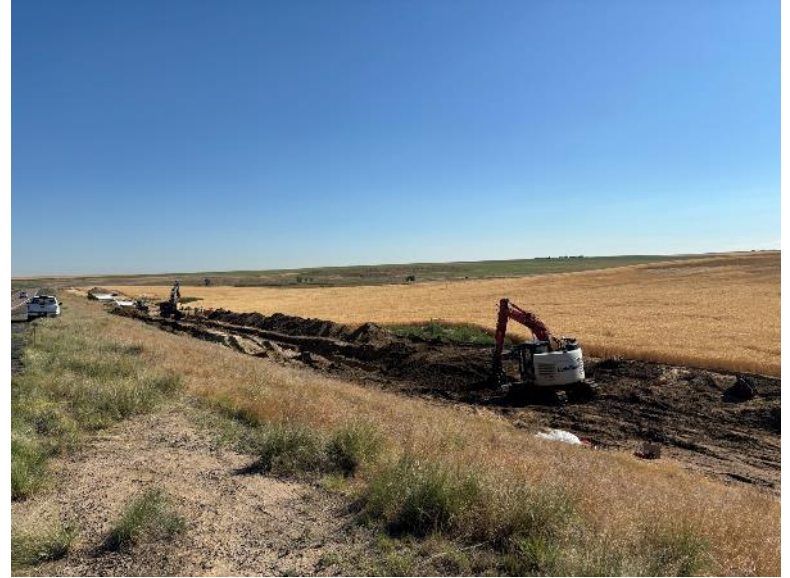
Construction crews install a portion of the DIA pipeline
