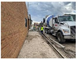
Work began with the ADA improvements downtown on Third St. and Jerry St. The Town's contractors are repairing damaged concrete in preparation for its scheduled surface treatment. Sidewalk, curb and gutter repairs are expected to run through May.
