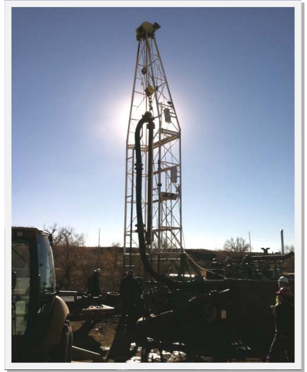
Castle Rock Water maintains an extensive network of deep groundwater wells. This picture shows the drilling of one such well.
