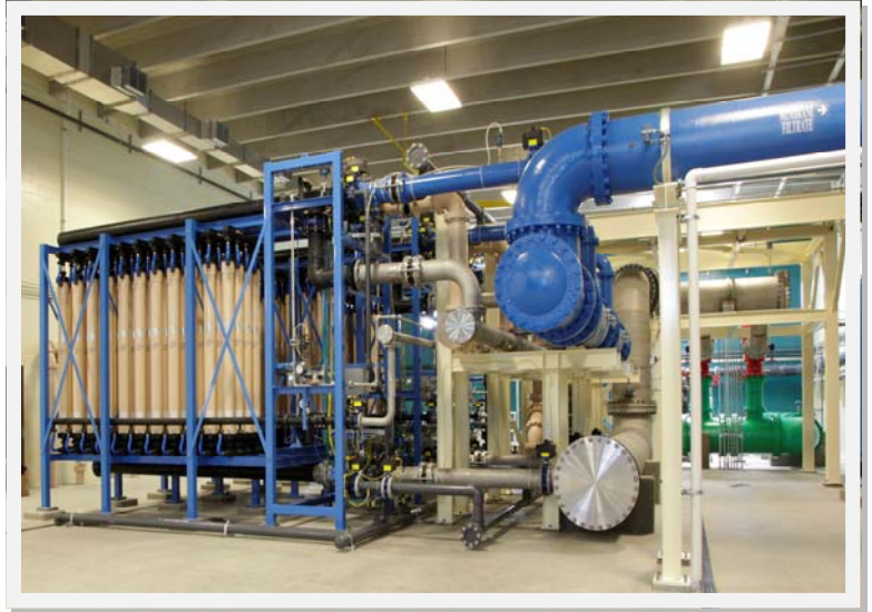
The membrane filters pictured above are the heart of our new Plum Creek Water Purification Facility.
