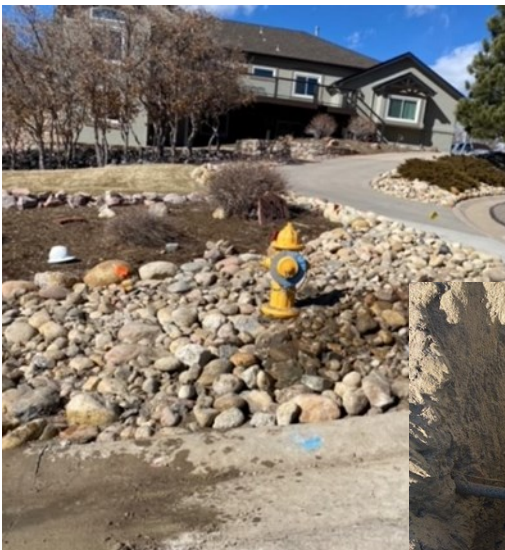
A leaking hydrant was replaced on October Place by the Distribution Team.
