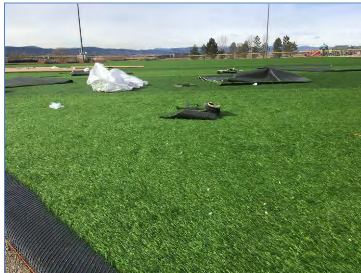
Installation of the artificial turf at the ballfields
