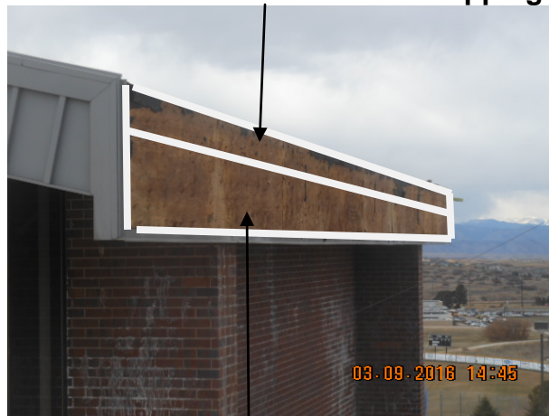
Ice & Water Shield over wood panels
