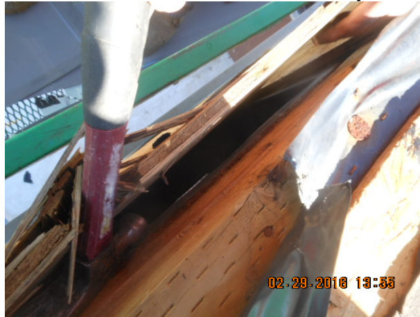
2" x 6" wood studs behind wood panels
