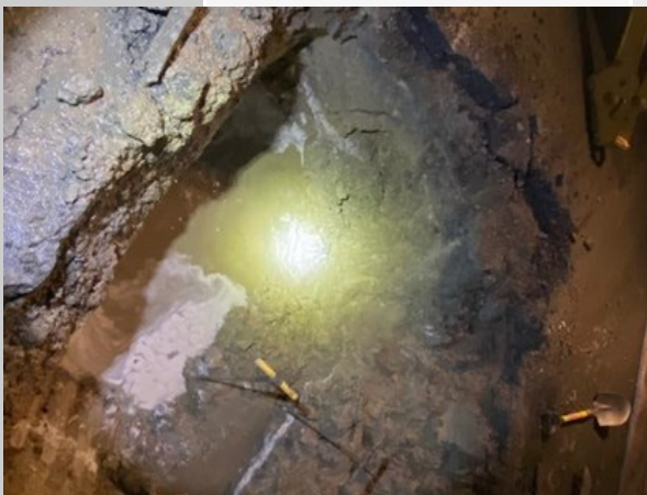
There was a main break in old town, staff was able to conduct the beam break repair on the 6" cast iron pipe. No residents were affected as this was conducted as a live repair.
