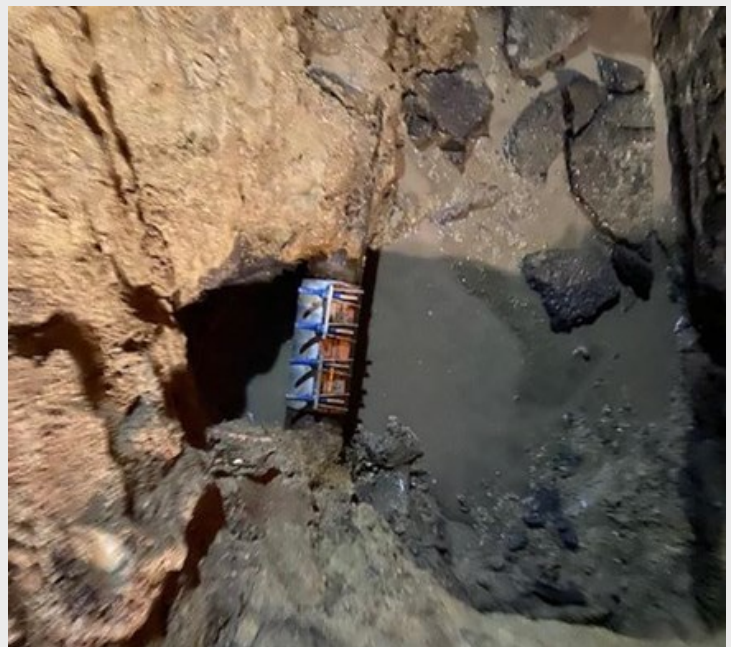
There was a main break in old town, staff was able to conduct the beam break repair on the 6" cast iron pipe. No residents were affected as this was conducted as a live repair.
