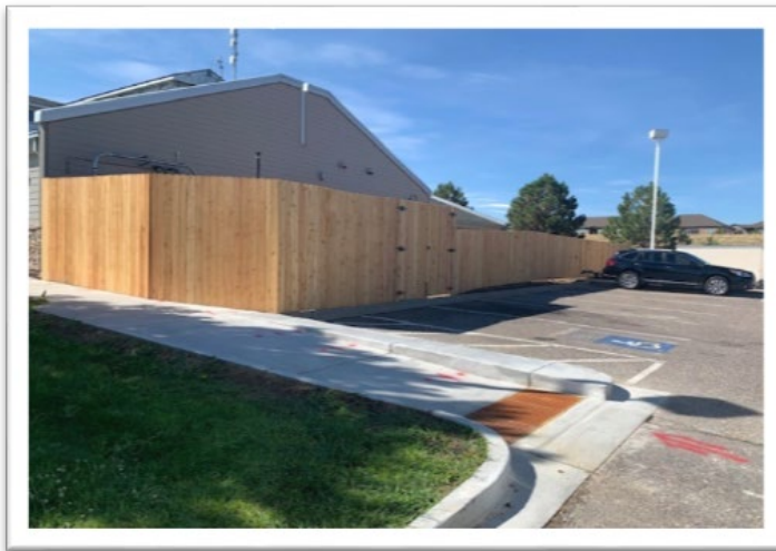
New fence and sidewalk at Station 154
