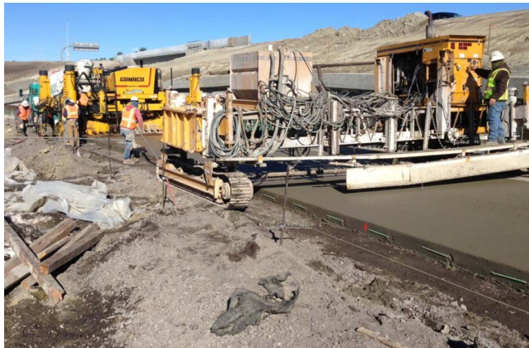
Concrete Paving I-25 Southbound On-Ramp
