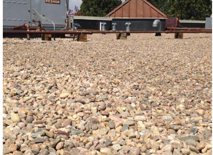
After the skylights were removed, the roof was patched and additional rock ballast installed
