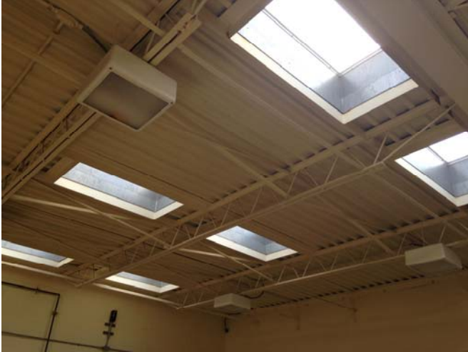
Pictures showing the many skylights in the filter bay at Meadows WTP before the new roof – most were leaking
