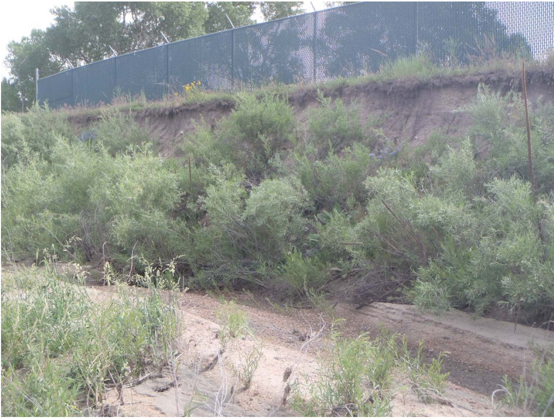
Looking northeast – bank erosion along well field fence.
