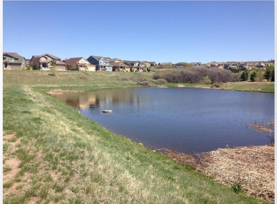
Existing Retention Pond
