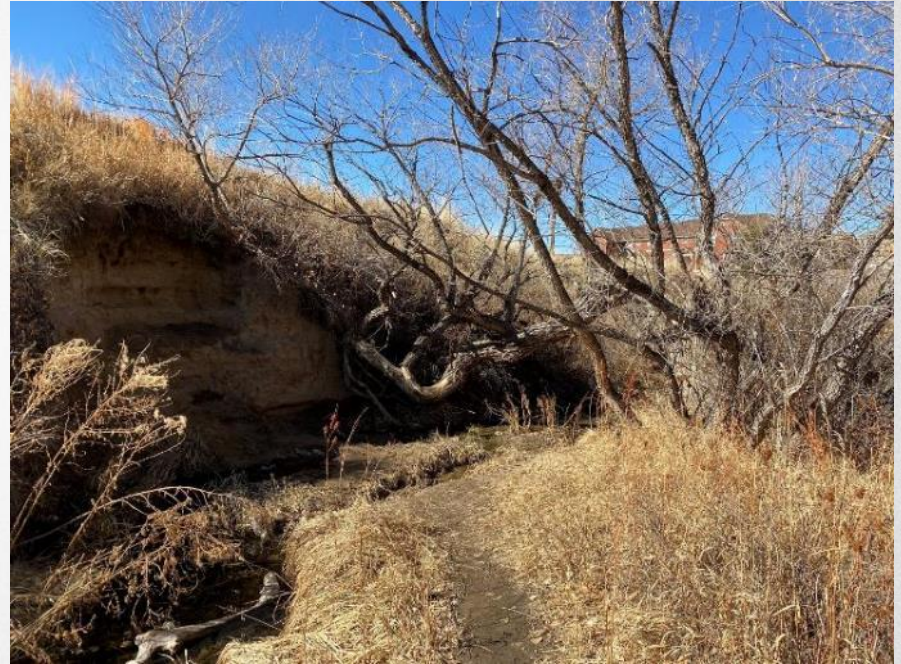
Bank Erosion adjacent to Paved Trail
