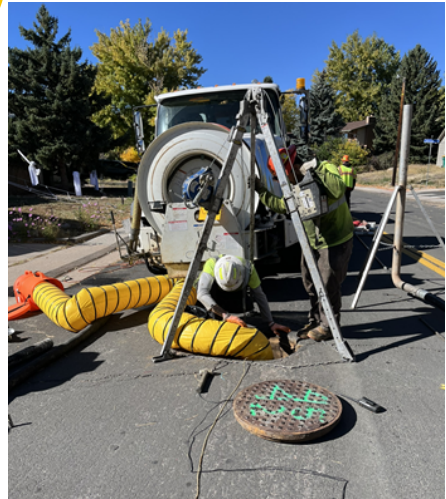
Contractor setting up confined space entry PPE on the downstream manhole so the crew member can climb into the manhole with the liner.
