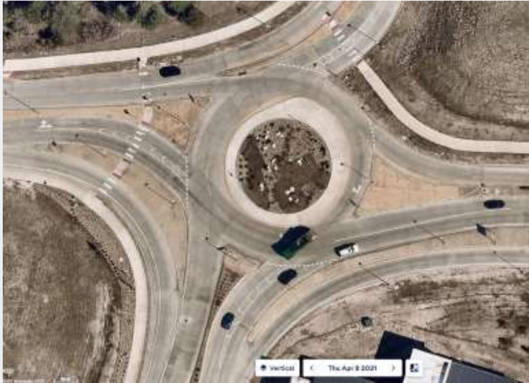
Before ground in thermo installed
