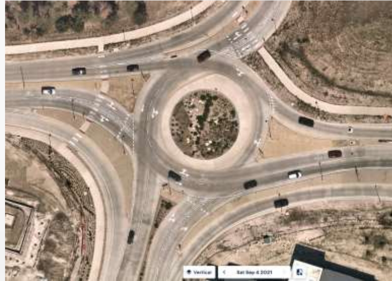
After ground in thermo installed
