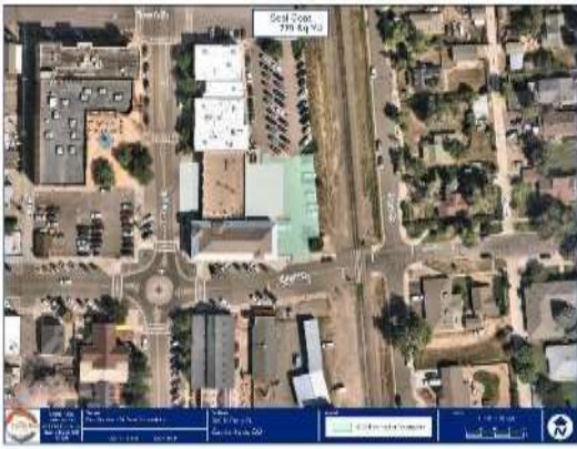
Perry St. Fire Station
