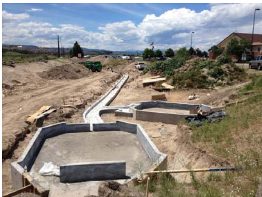
Recently poured concrete forebays and trickle channel
