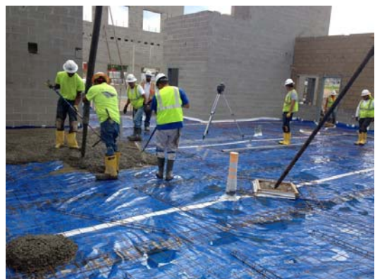
Crew pouring concrete slab-on-grade in the building
