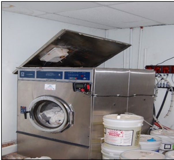
Dryer where a fire originated
