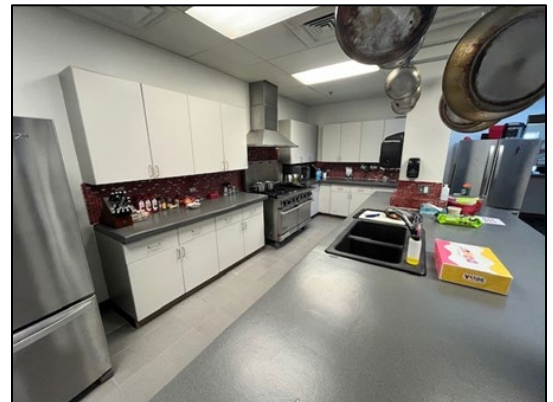
Station 154 counter top refinish
