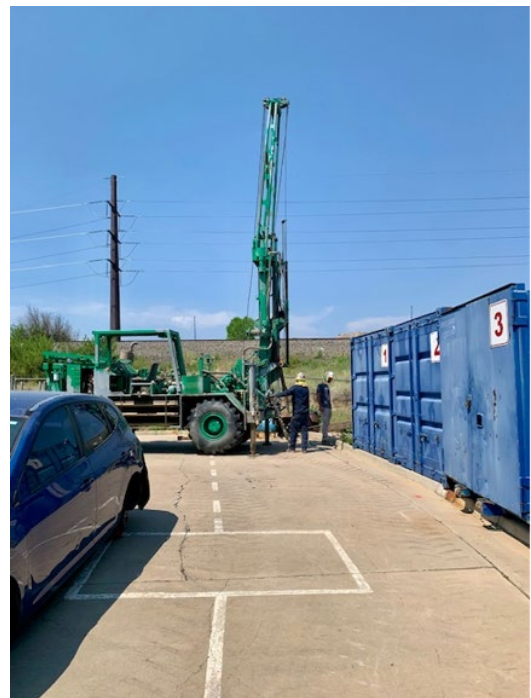
Soil Sampling at the tower
