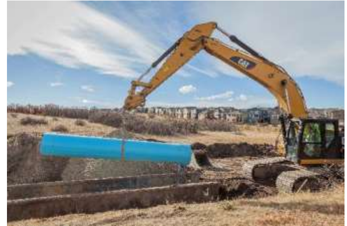
Section of 36 inch PVC pipe being lowered into trench
