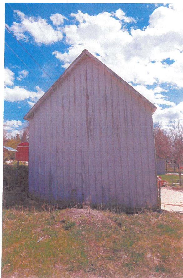
Photo 7 Barn – North Side, camera facing south
