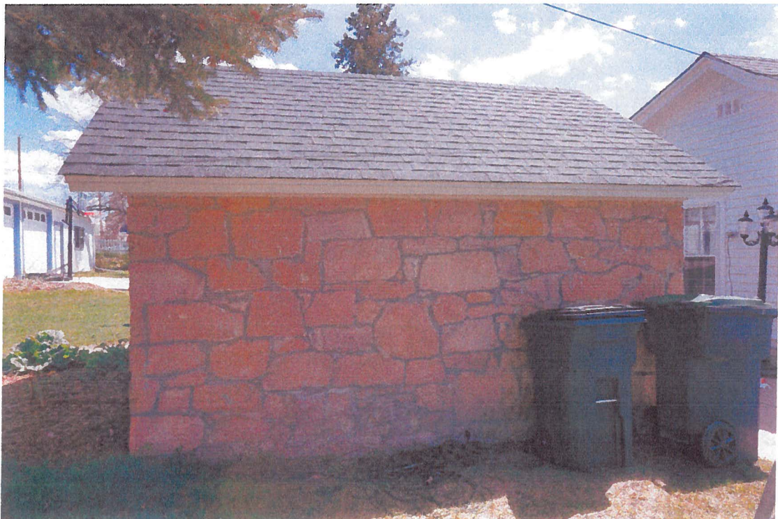
Photo 14 Ice House – North Side, camera facing south
