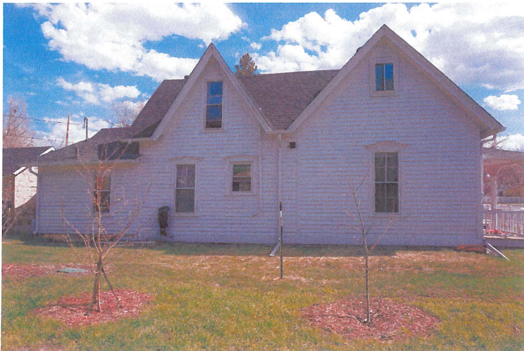
Photo 4 House – North Side, camera facing south
