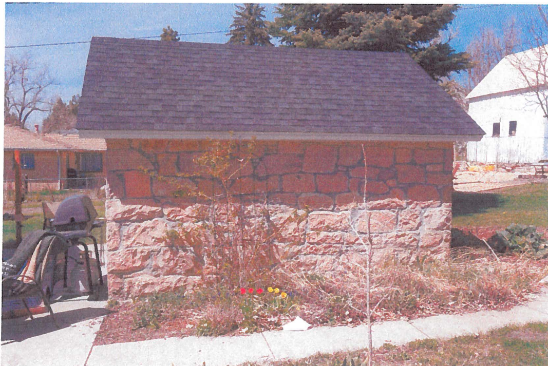
Photo 12 Ice House – South Side, camera facing north
