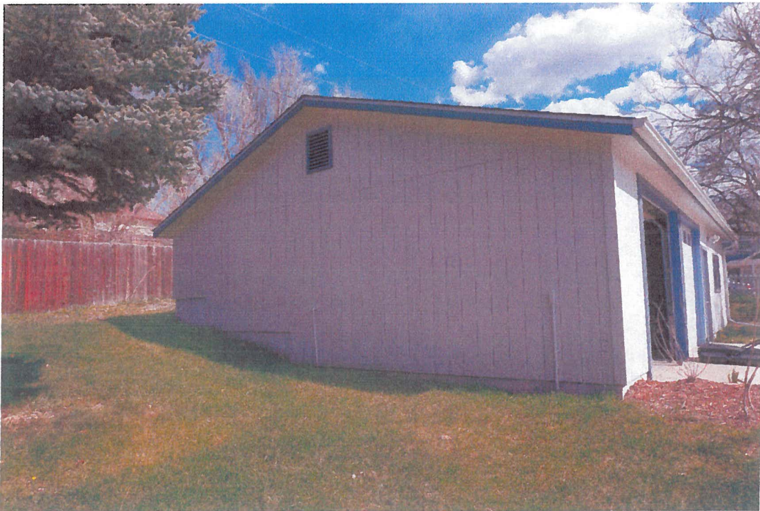
Photo 18 Garage – North Side, camera facing south
