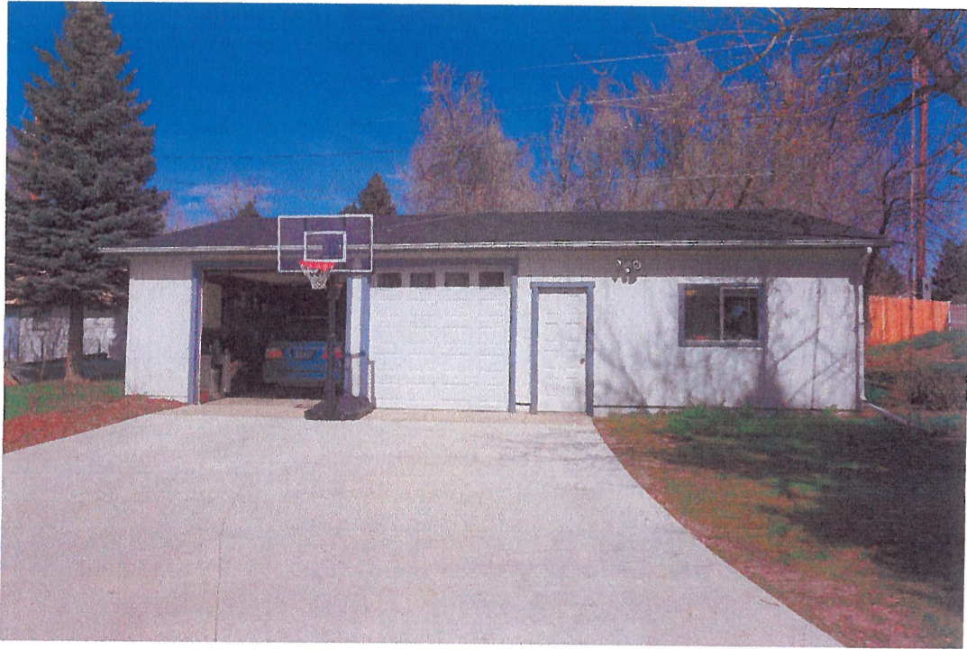
Photo 15 Garage – West (main) Façade, camera facing east
