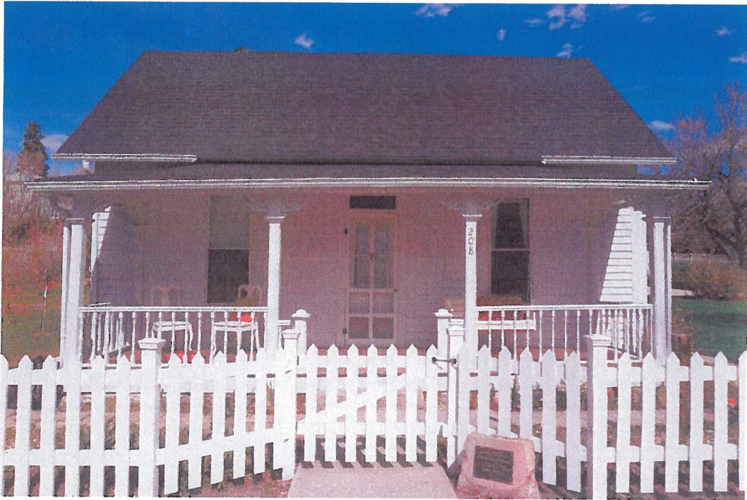
Photo 1 House – West (main) Facade, camera facing east
