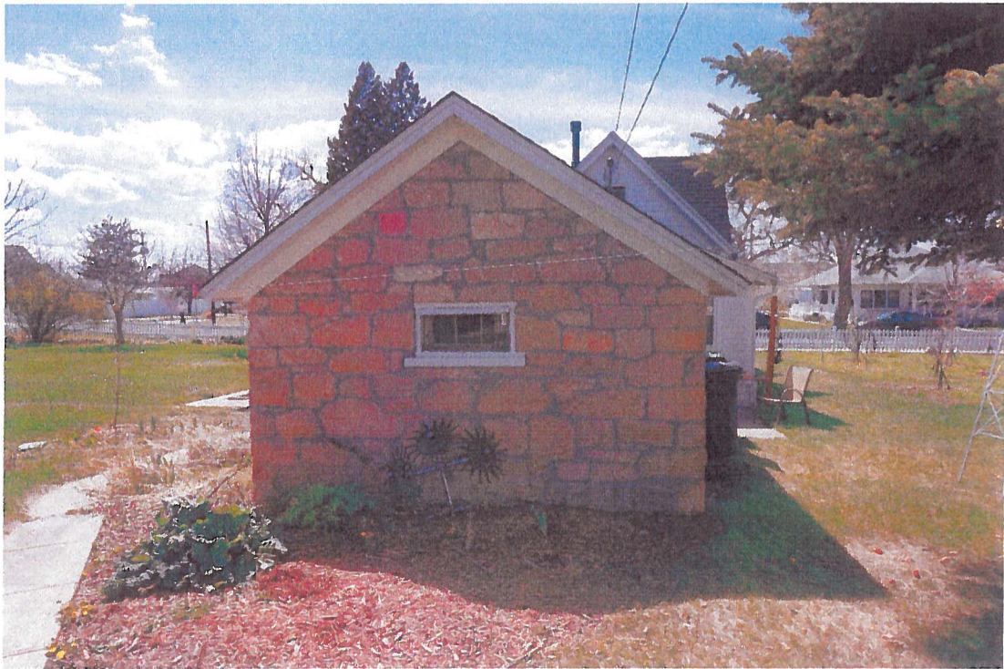
Photo 13 Ice House – East Side, camera facing west
