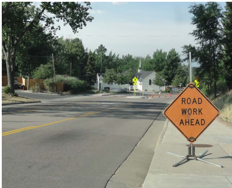
Street Maintenance Work on 5th Street
