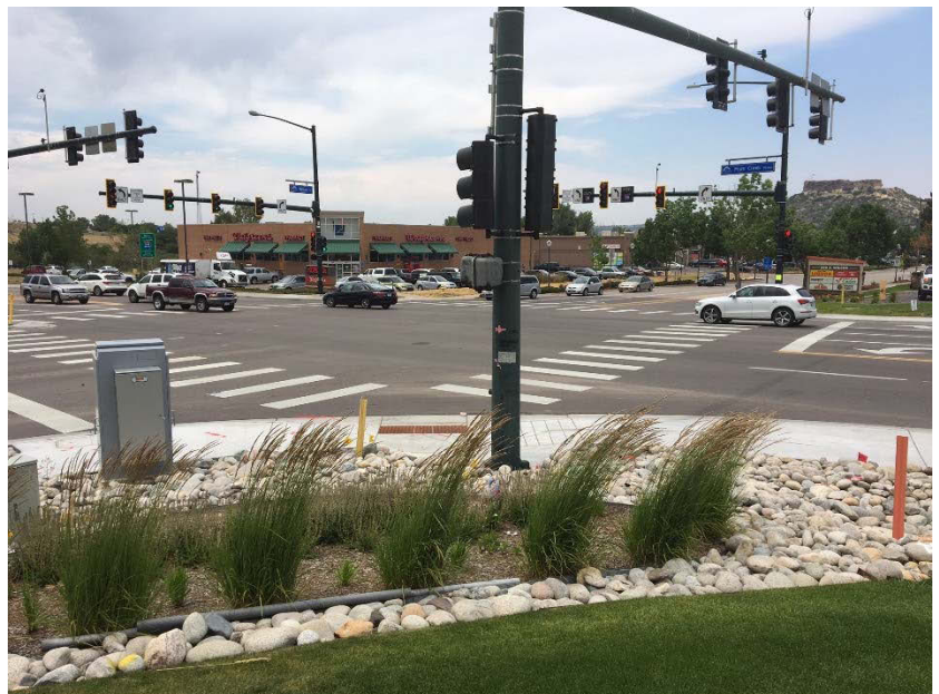
Completed Improvements at Plum Creek Parkway and Wilcox Street
