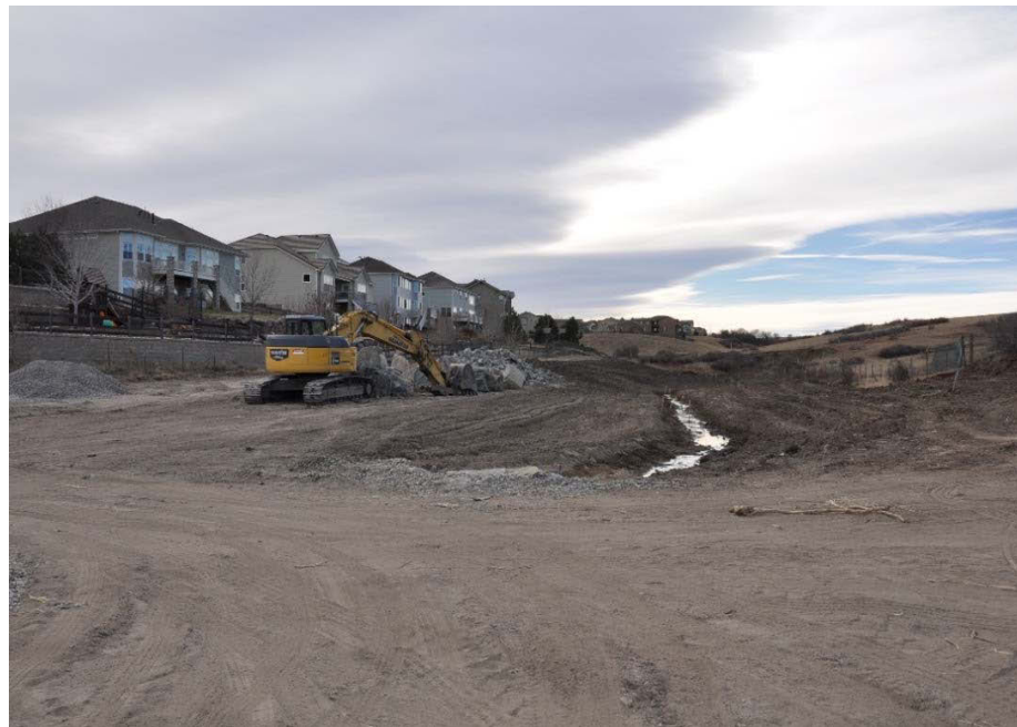
Tributary Stabilization Project in Progress
