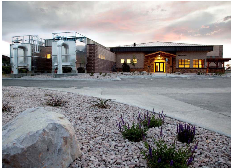
Plum Creek Water Purification Facility
