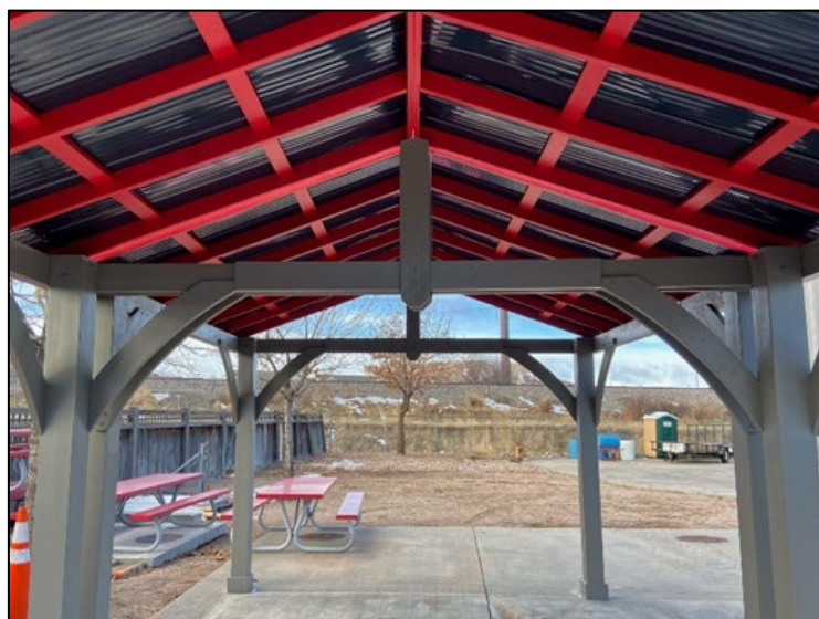
FTC weather shelter improvements
