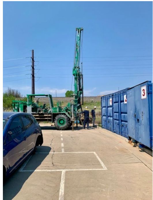
Soil Sampling at the tower
