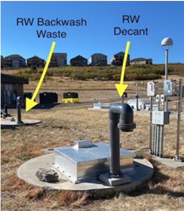
In response to new regulations regarding facility venting, the plant maintenance team installed new “candy cane” style vents at Ray Waterman WTP and Tank 9.
