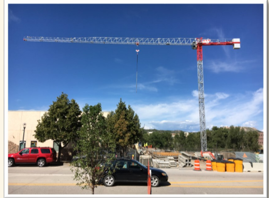
Riverwalk Project Progress August 24, 2017
