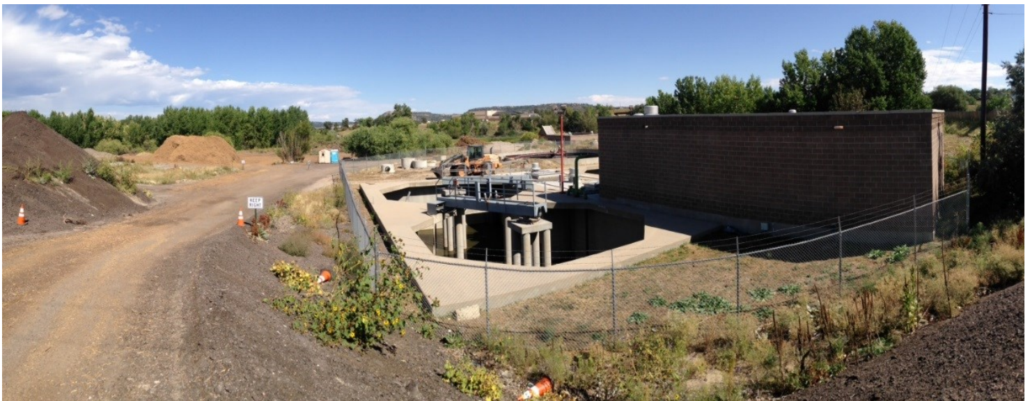
Old wastewater treatment plant before demolition – Sep. 13, 2017.
