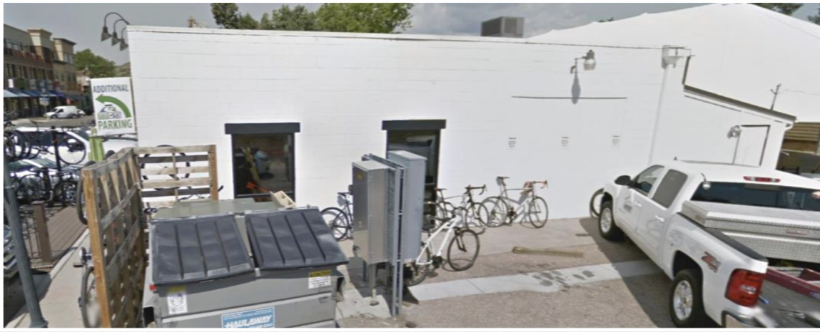
Existing View of East Side of Building
