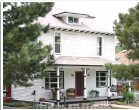
Existing Front Façade
