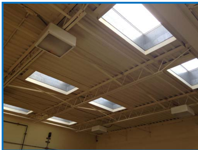
Pictures showing the many skylights in the filter bay at Meadows WTP before the new roof – most were leaking
