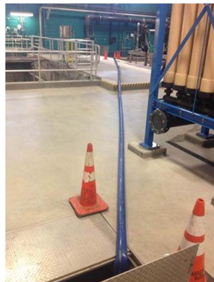
Pumping down the membrane feed well
