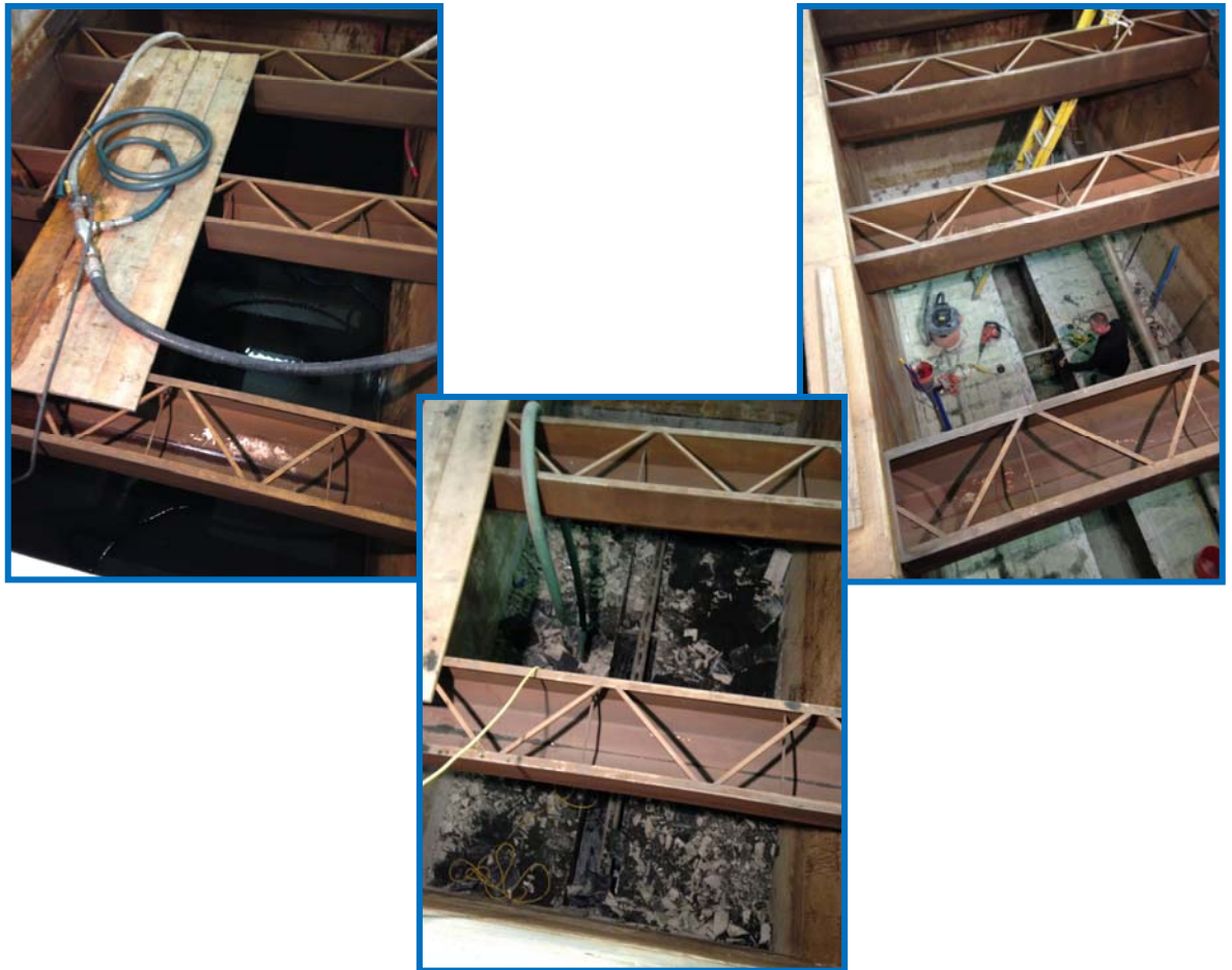
Showing three stages – vacuum media out, demo underdrain & remove, and prepare base, filter gullet and air scour piping for new underdrains.
