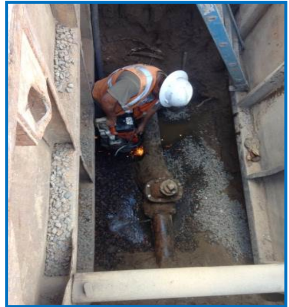
Cutting valve out to install new valve
