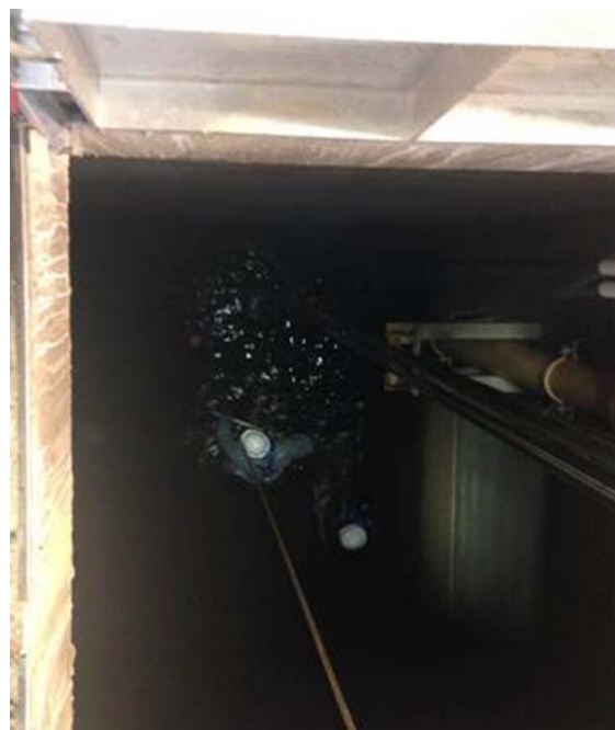
Removing sediment from the recycle basin
