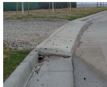
Curb ramps of earth, concrete, or lumber are not permitted in the curb section.
