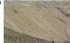
Erosion control blanket protecting a slope.
