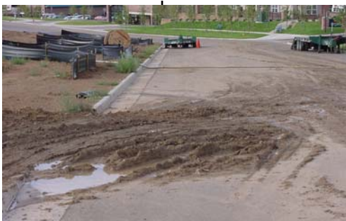
DON'T No vehicle tracking control means mud on streets and an immediate Stop Work Order.
