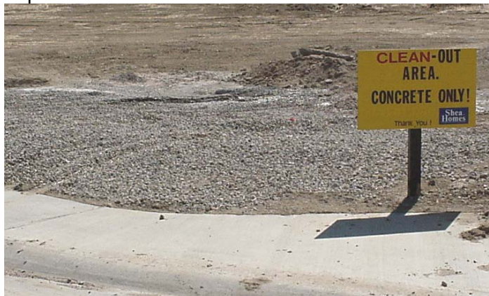
DO A properly installed concrete washout area with Vehicle Tracking Control.
