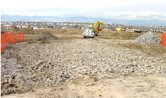
DO Properly installed vehicle tracking control.
