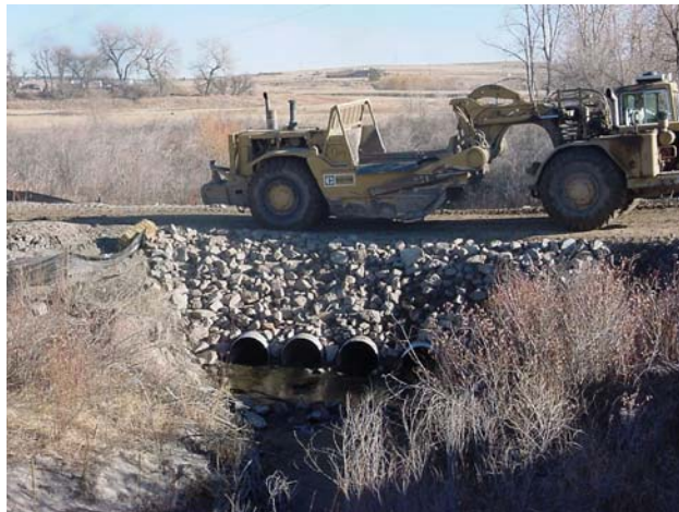
DO Properly installed temporary stream
