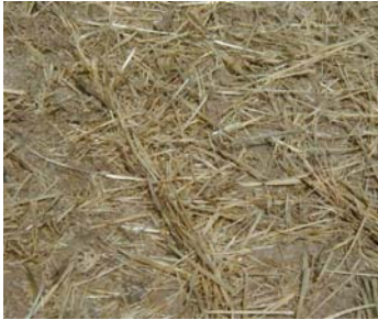
Seeding and mulching (SM) reduces erosion and is considered an erosion control.
