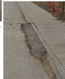
Curb ramps of earth, concrete, or lumber are not permitted in the curb section.
