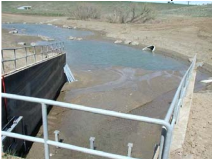
Sediment that accumulates in water quality ponds needs to be cleaned-out periodically, requiring significant effort and cost.
