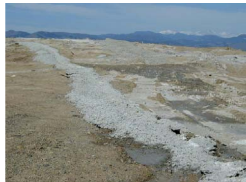
DON'T Extensive wasting of concrete on the construction site requires additional effort to clean up and can impair subsequent revegetation operations.
