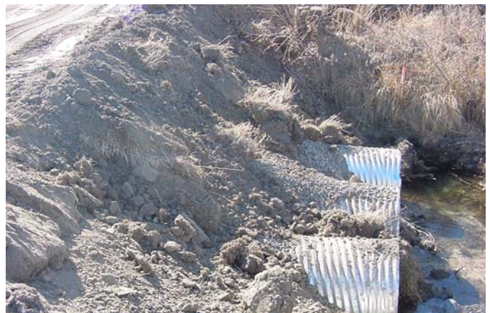
This temporary stream crossing is constructed of soil and is not acceptable.
