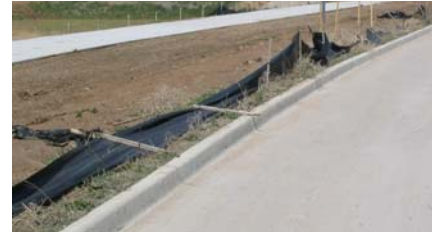
Silt fence should be located far enough off streets to avoid damage from snow-plowing operations.
