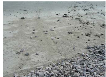
DON'T Use of low density rock such as Rhyolite is not permitted since it does not stay in place and can get tracked onto paved streets.
