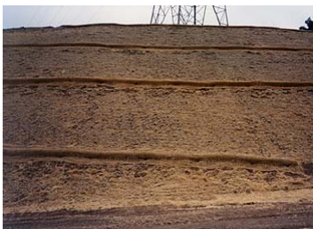
A sediment control log (SCL) captures eroded sediments and is considered a sediment control BMP.
