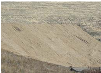
Erosion Control Blanket (ECB) shall be used on slopes greater than 4:1.
