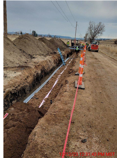
Pipeline and conduit installation in Walker Road
