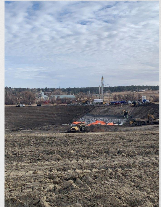
View of the reservoir run-down with well drilling rig in background
