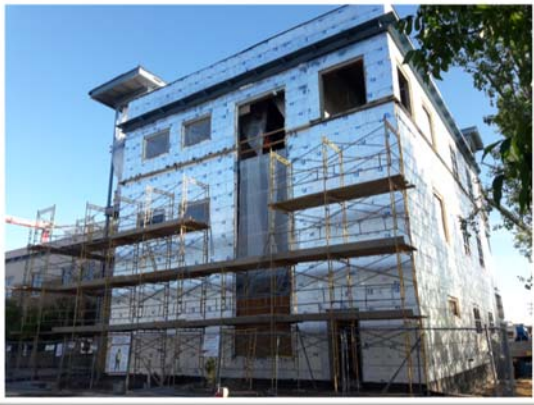
Town Hall Addition July 28, 2017
