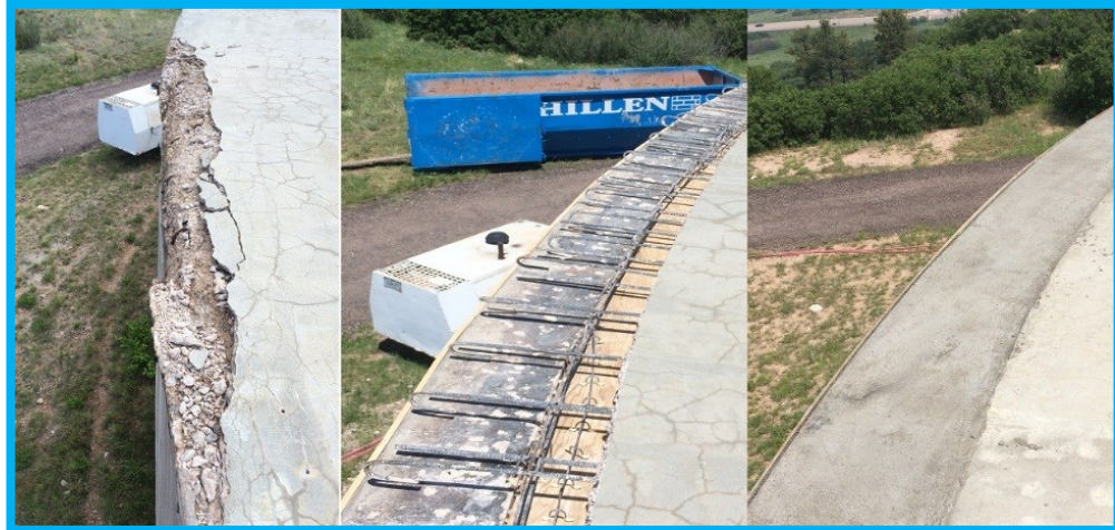
Tank 3 Concrete Roof Repair Sequence
