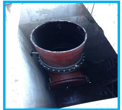
Left to right: Cutting and removing the 20,000 plus pounds of concrete; reinforcing and formwork for new concrete beam and hatch curb walls; and the new 42" diameter ductile iron pipe system.
