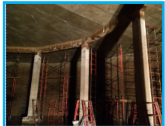
Tank 3 Temporary Shoring
