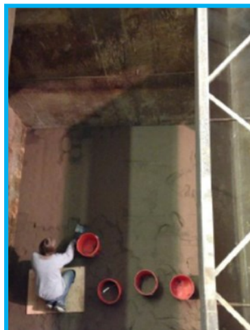
Skimming Fines off Media Layers during Installation
