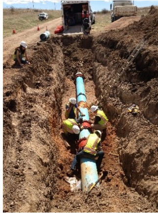
A repair was made to a broken 16" raw water line which feeds water from the North Central Well Field to the water treatment plant. A total of 26 feet of pipe was replaced.
