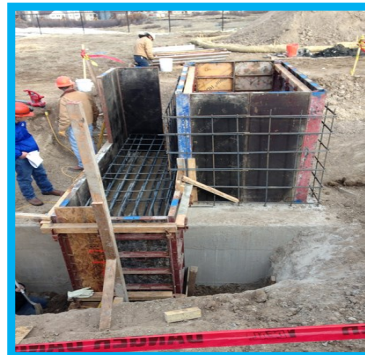
Left to right: Cutting and removing the 20,000 plus pounds of concrete; reinforcing and formwork for new concrete beam and hatch curb walls; and the new 42" diameter ductile iron pipe system.
