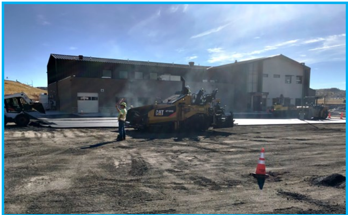
Asphalt Work at the O & M Building
