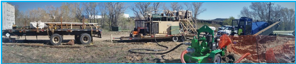
Well CR-12R Drilling
