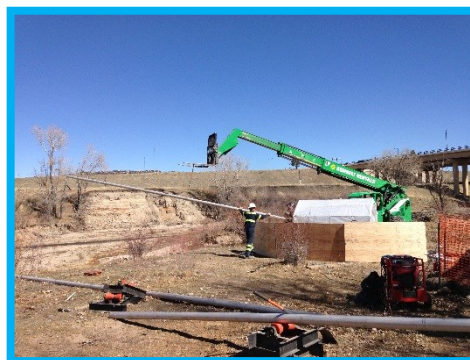
AL-16 Lateral Arm Installation
