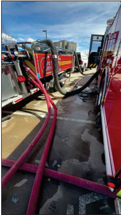
Pump testing with the Draft Commander
