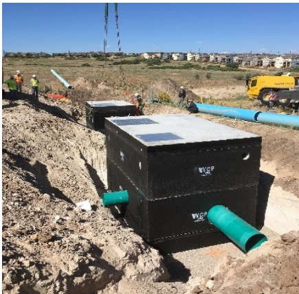
Meter and flow control vaults being installed near the RWRWTC.
