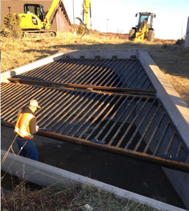
Grates were also installed on stormwater pipe in this area to improve public safety.
