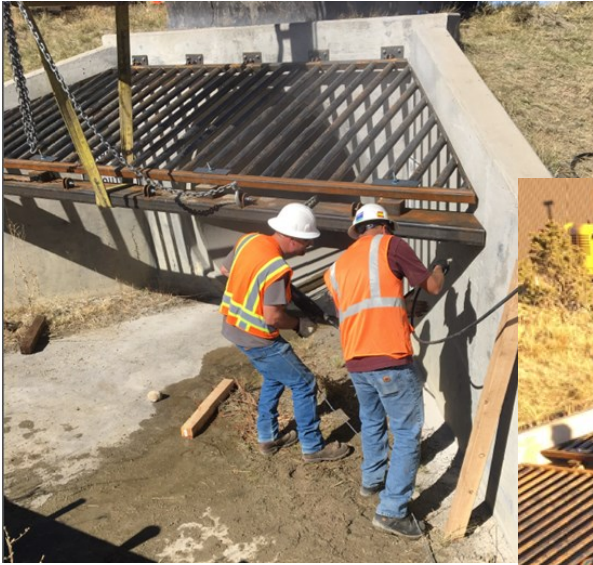
Grates were also installed on stormwater pipe in this area to improve public safety.
