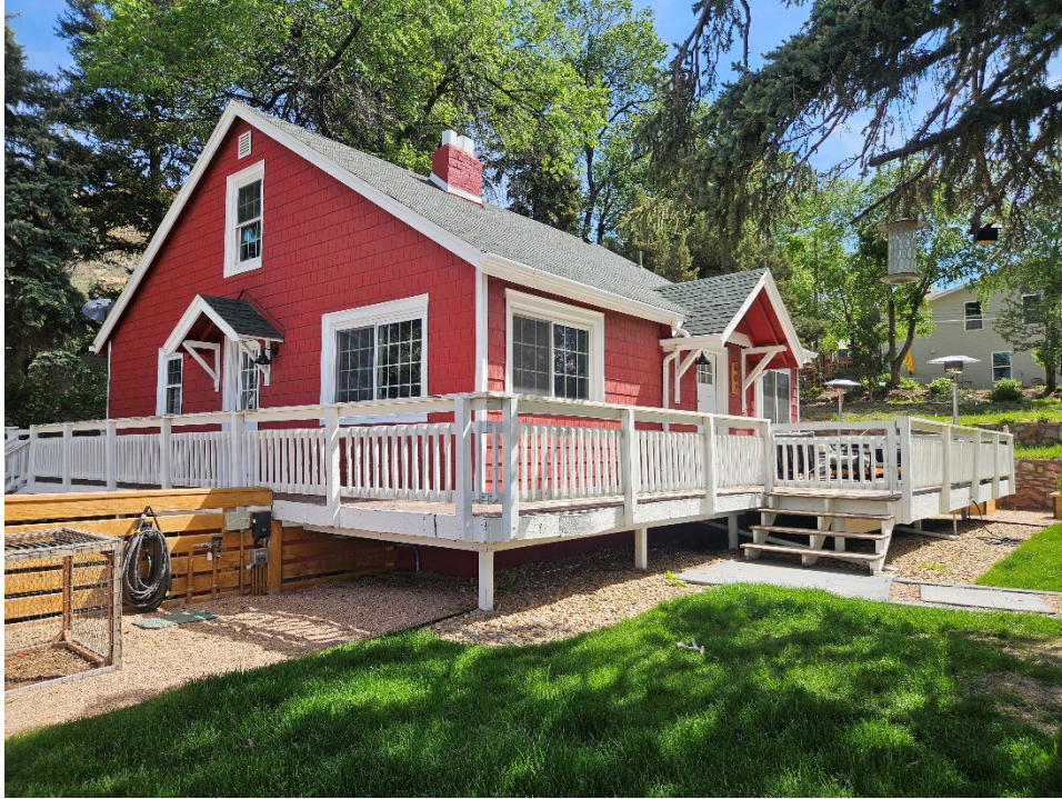
Primary (south) and west elevations of the residence, view northeast (Roll 26-450, image 103604; Emily Wren; 5/22/2026)
